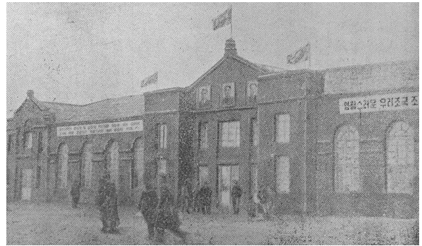
Figure 9. Newly Built Temporary Pyongyang Station (source: The Rodong Sinmun , 1954, January 13)
