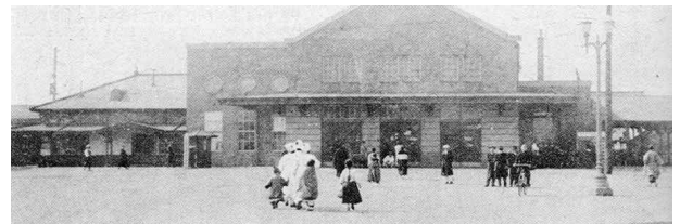
Figure 3. A New Addition to the front of Pyongyang Station, under construction, 1940 (source: History of Transportation in Joseon , 1986)
